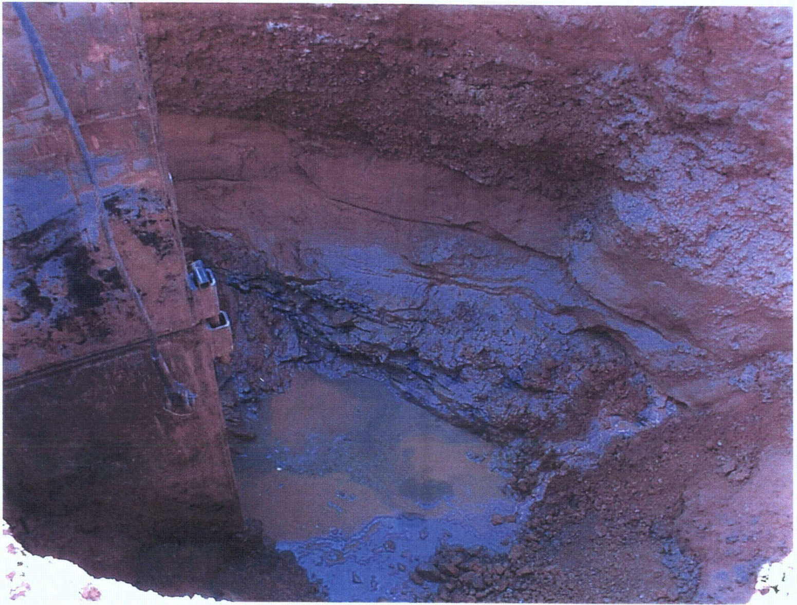
Figure 3. Water entering the excavation (concrete riser pipe location) at the interface of sandy soil and black shale.
