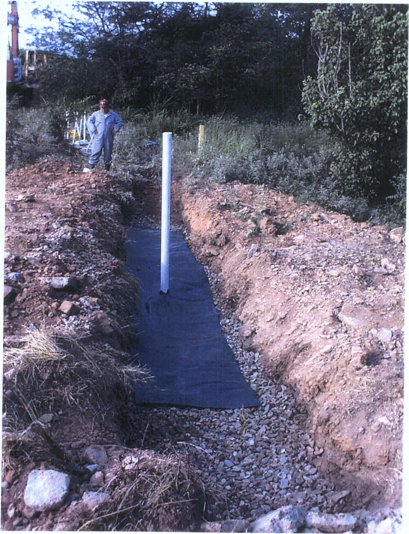
Figure 9. Monitor trench construction. (Looking South)
