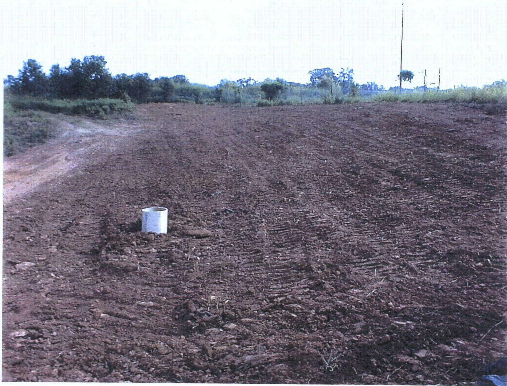
Figure 8. Final grade of area with riser pipe showing. (Looking North)
