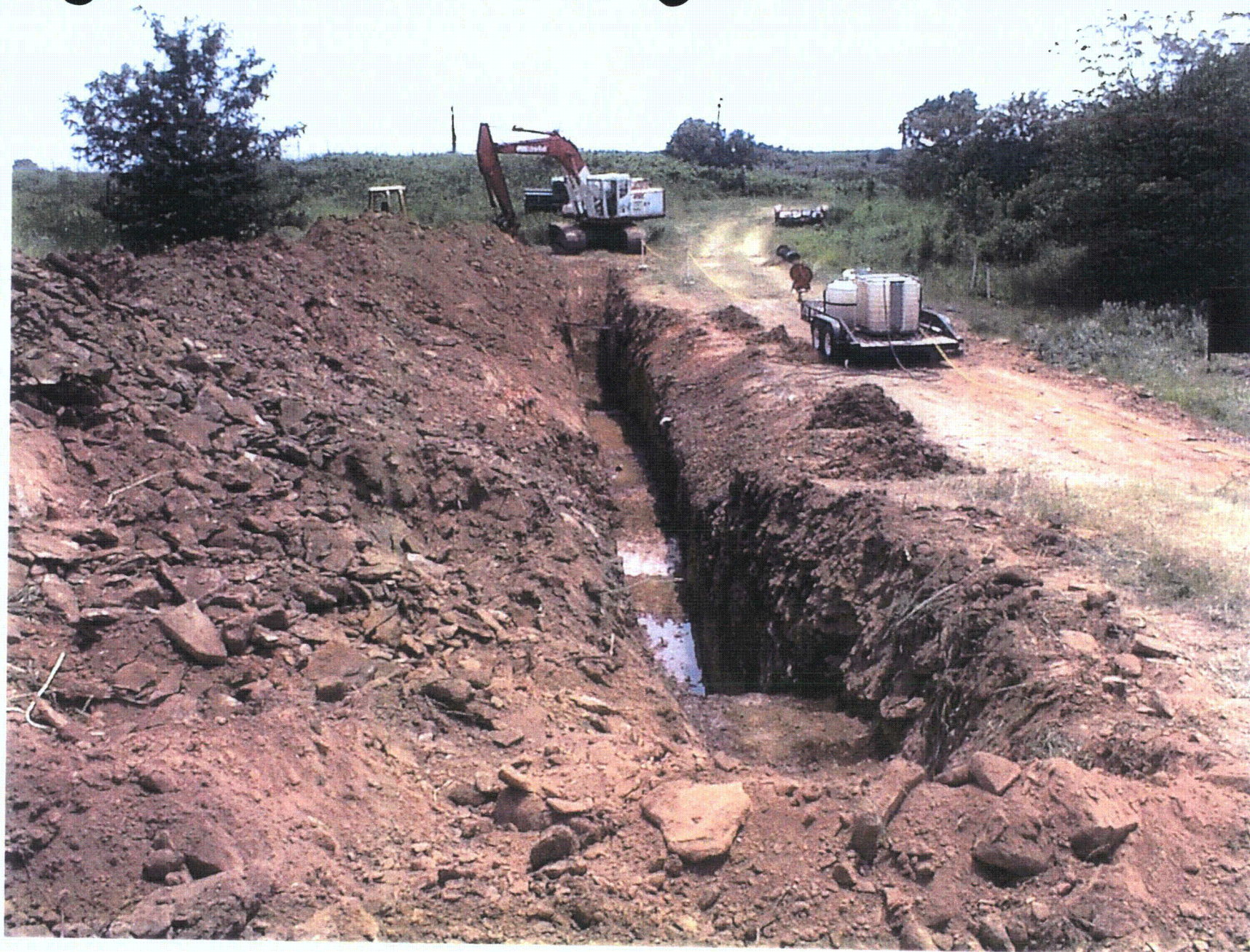
Figure 1. Open trench excavated to the top of sandstone. (Looking South)
