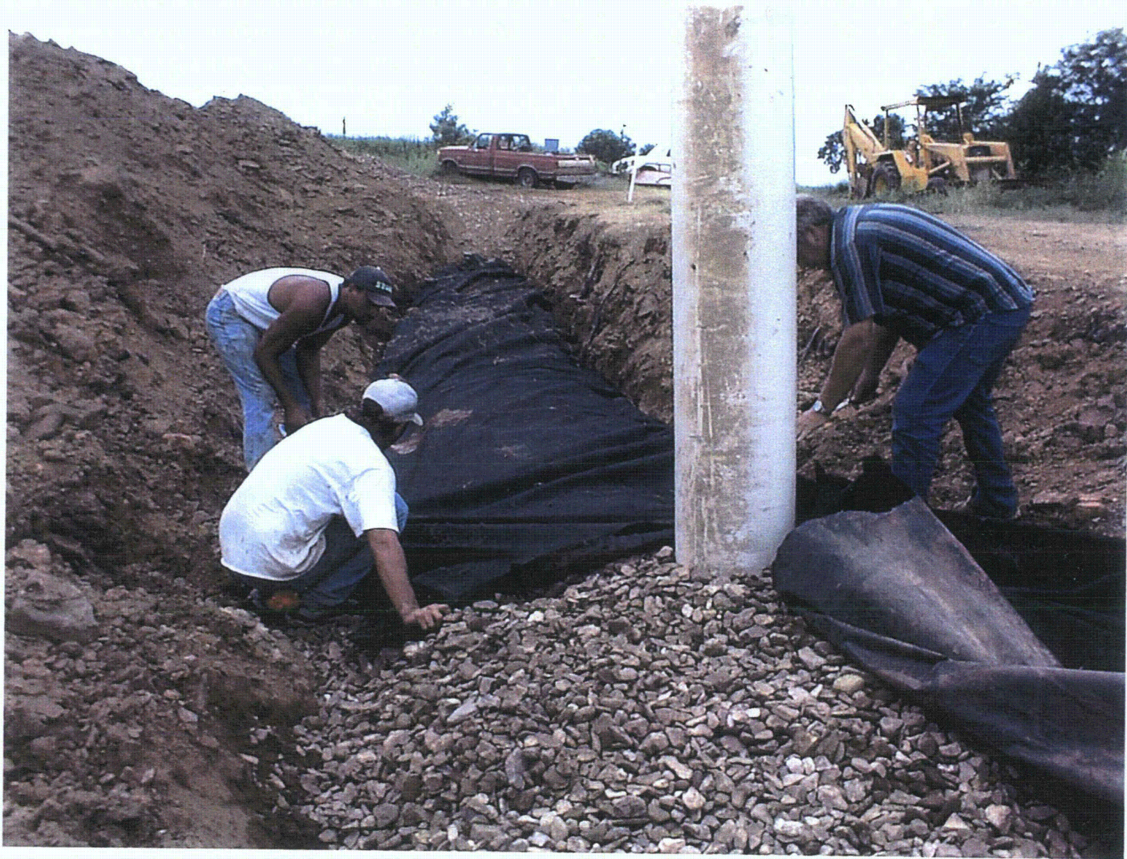
Figure 7. Placement of liner and geo-fabric over gravel. (Looking South)
