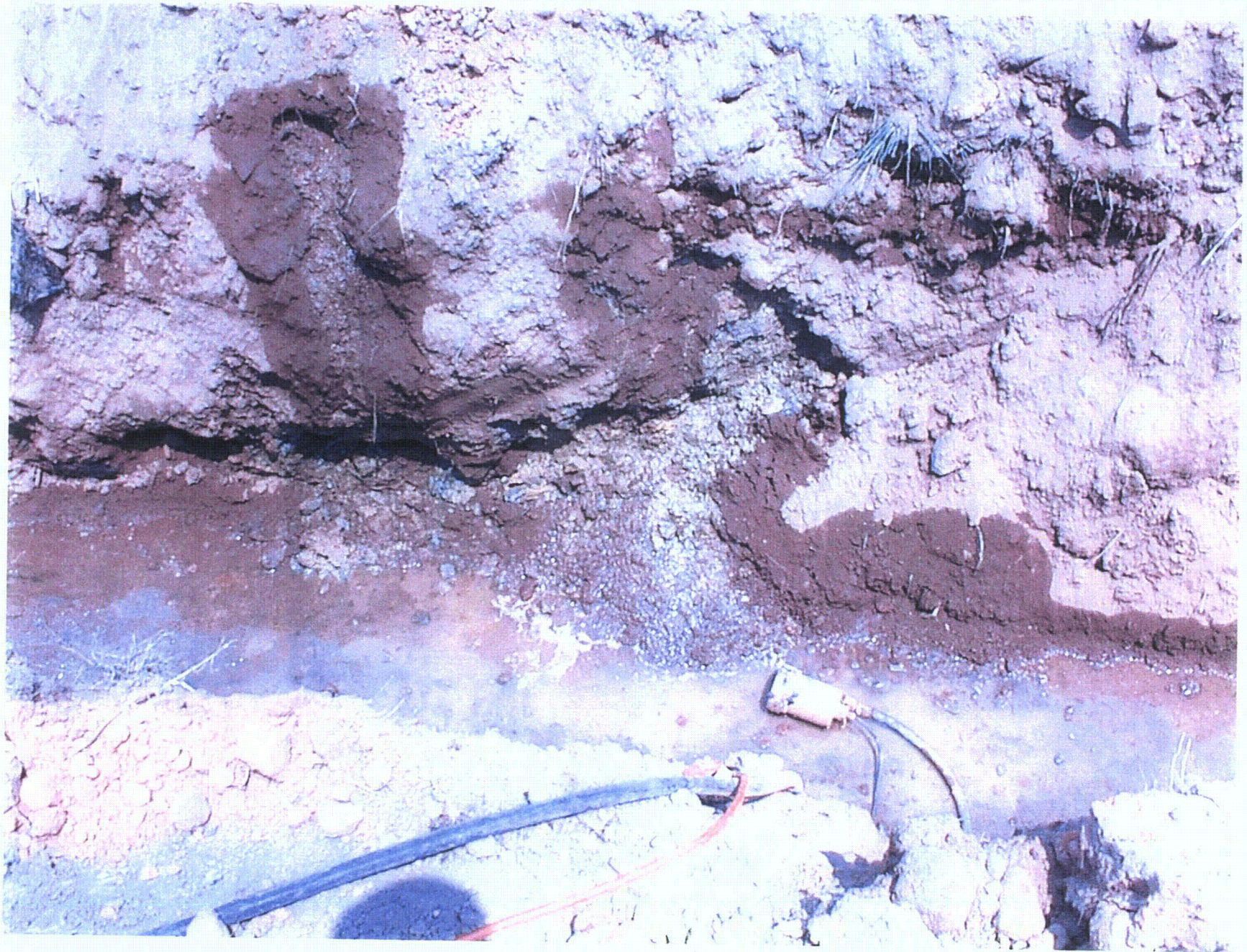
Figure 3. Seepage from east wall of trench - riser pipe placed at this location.
