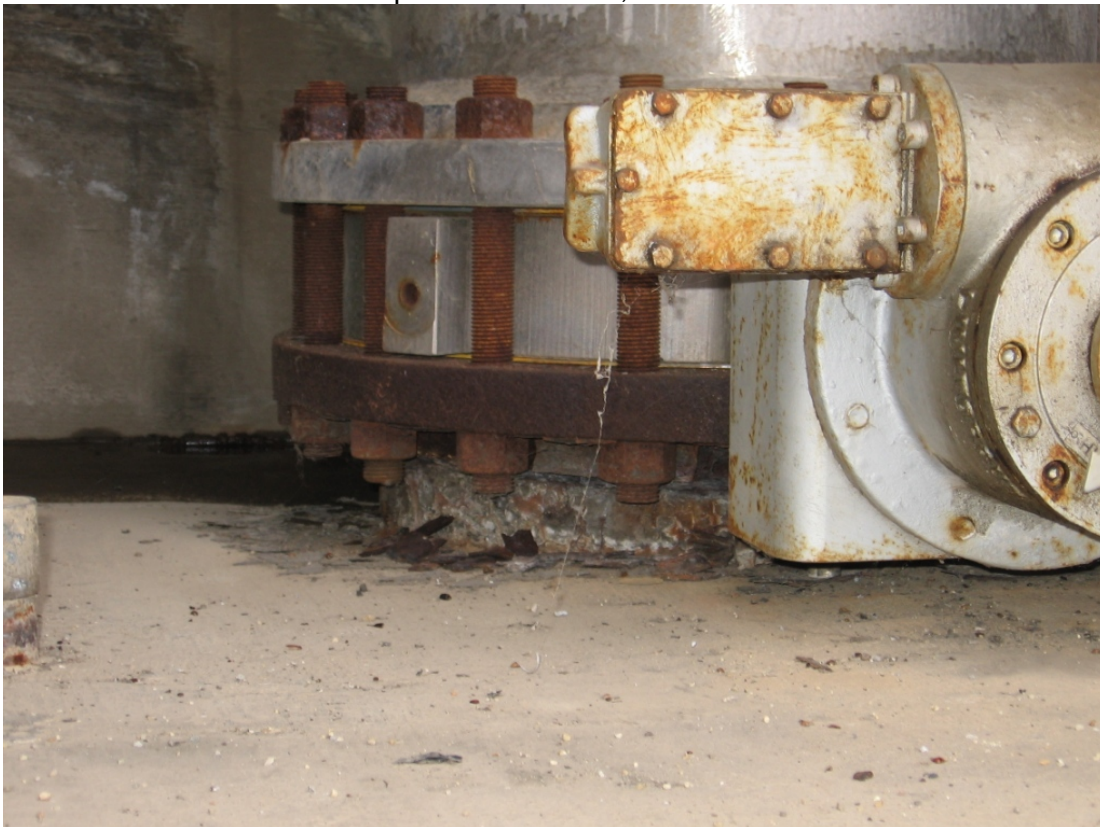
Picture No. 2 - 0B SX Riser Pipe- November 30, 2006
