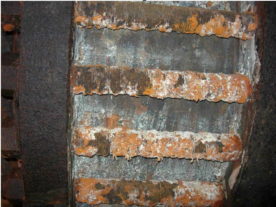
Picture No. 8– 0SX 138B Valve Bolting - October 2007
